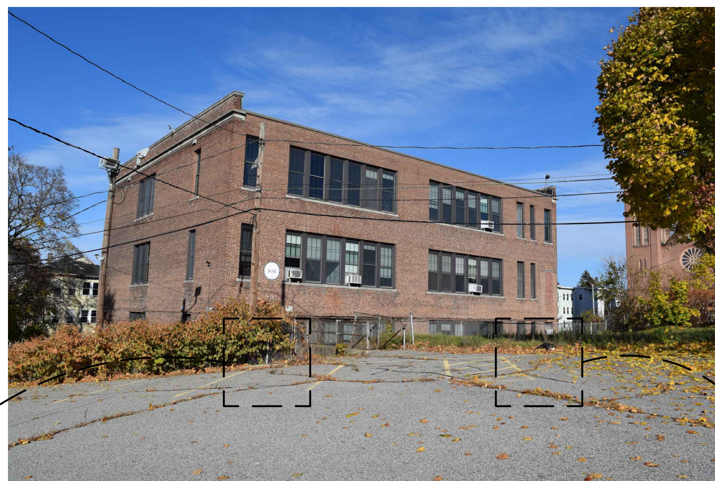
SOUTH ELEVATION VIEWED FROM EXISTING PARKING LOT
