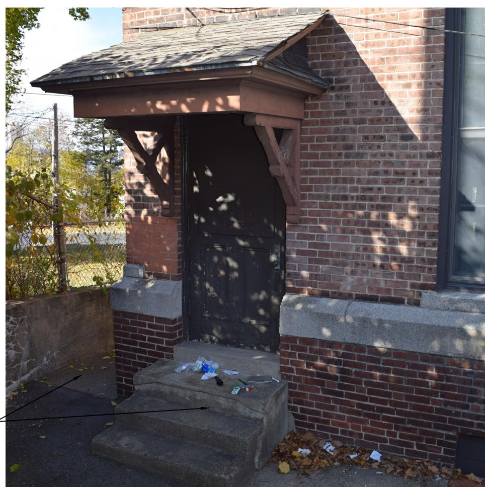
DOOR AT SOUTHWEST CORNER - TO BECOME THE MAIN ENTRANCE
